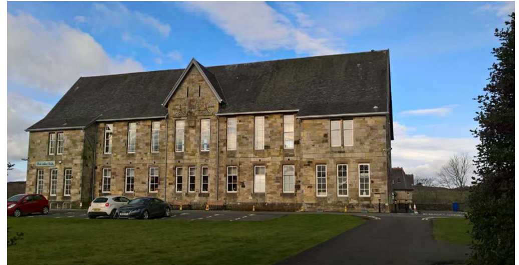
The Canadian Garden sits in front at the south of Sommerville Weir Hall
