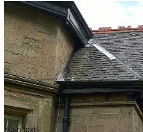
Overlaid zinc flashing over original lead
