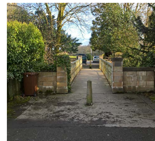
Footbridge linking Faith Avenue to Peace Avenue
