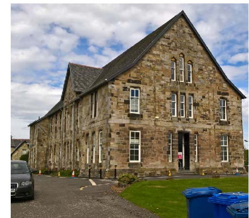
Sommerville Weir Hall - The Central Building
