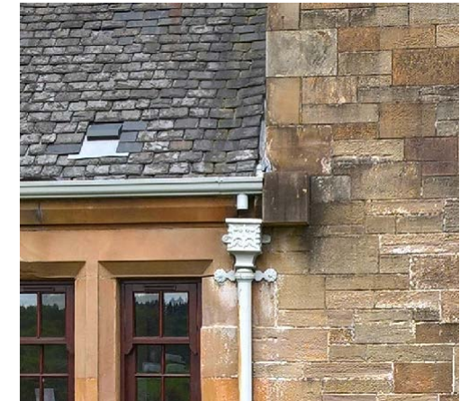
Original cast iron fittings at Glenfarg
