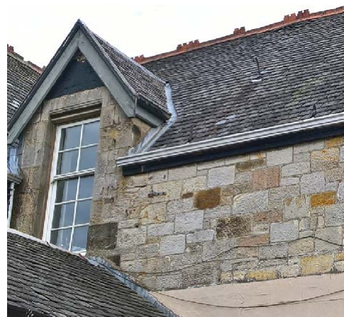
Replacement guttering in aluminium
